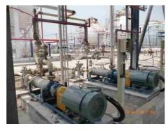
SC MAG-M65 / 5 stages, for pumping of ISOBUTYLENE Q=35 mc/h, H= 40m; Ningbo - China.
