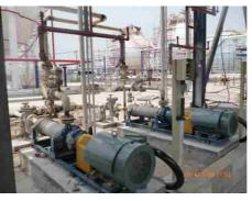
SC MAG-M65 / 5 stages, for pumping of ISOBUTYLENE Q=35 mc/h, H= 40m; Ningbo - China.
